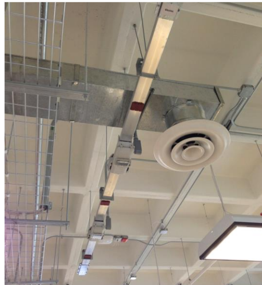
POWER SERIES – COMPACT AIR INSULATED 100A – 1250A
